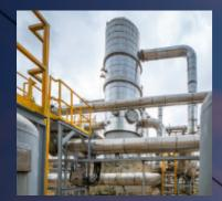
Kaishan ORC Screw Expander uses an organic medium such as working fluid; preventing the use of diesel or gasoline during operation, and achieving thermo technical conversion without emission, consumption, or pollution. The power generated by the plant can be directly connected to the power grid when the original power supply and operation methods are maintained, making our technology genuinely green and environmentally friendly.
